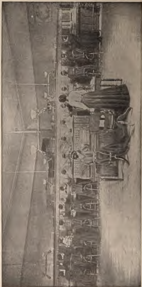
FIG. 159.—An Independent Telephone Exchange at Newark, N. J., equipped with the multiple transfer system of the Western Telephone Construction Co.
